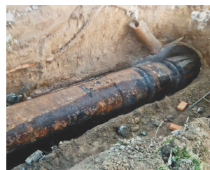
Fig. 2. Repair of pipelines using a traditional pipe method
