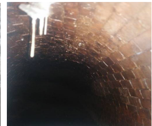
Fig. 4. Sewers built of clinker brick in Kharkiv
