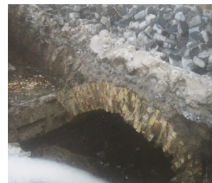
Fig. 3. Sewers built of clinker brick in Kyiv
