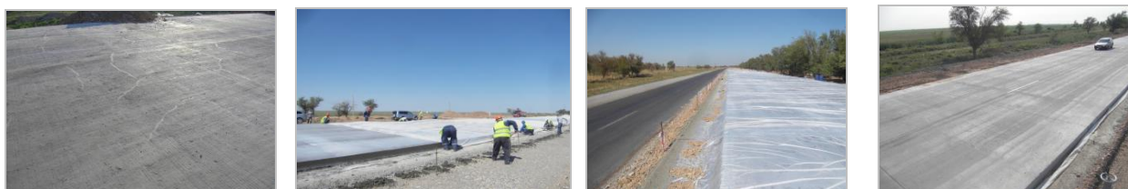
Fig. 6. Process of the curing test using polyethylene film
