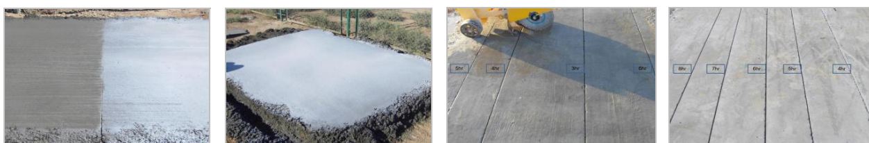
Fig. 2. Process of experiment (spraying the concrete curing compound and cutting joints)
