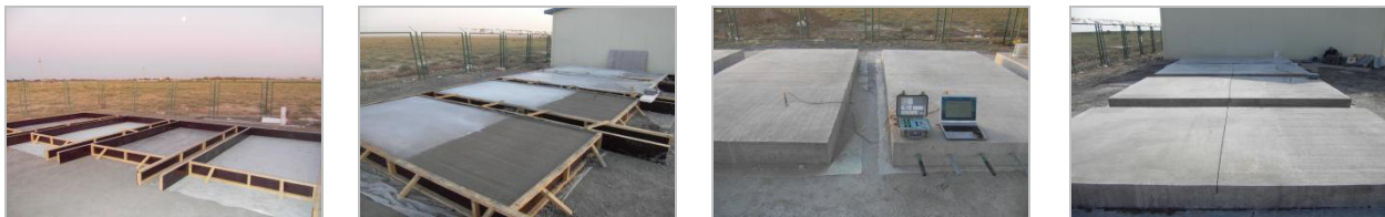
Fig. 3. Process of concrete slab mock-up test
