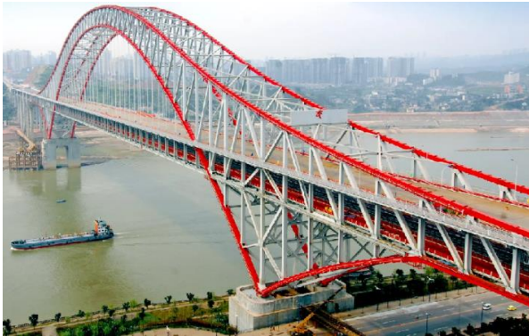
Illustration 6.1. Arched bridge trusses with traffic in the middle The support reactions of arched trusses are defined in the same way as
