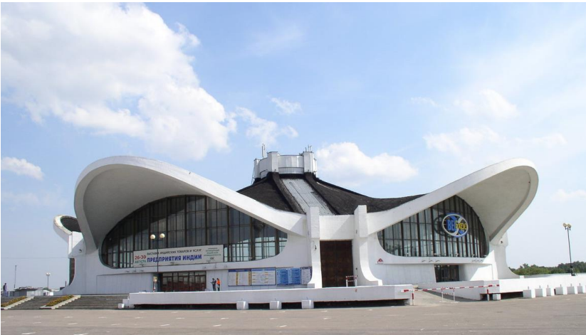
Illustration 1.2. Hanging shell of negative Gaussian curvature on an arched support contour
