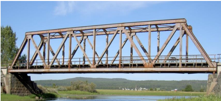
Illustration 5.1. Single-span bridge girders
