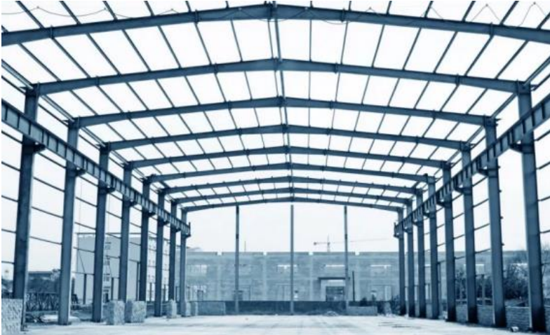
Illustration 8.1. Cross frames of the production building
