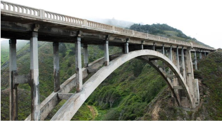
Illustration 1.4. Space system in the form of statically indeterminate arches with a beam over structure
