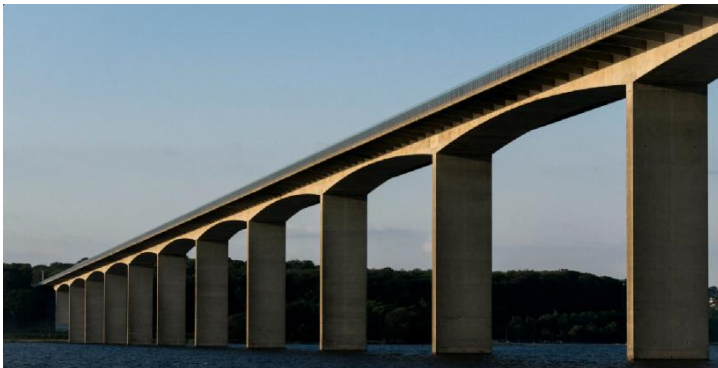
Illustration 1.5. Non-thrusting multi-span statically indeterminate beam with variable cross section
