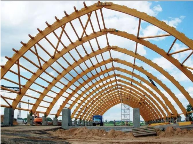
Illustration 4.1. Construction of a hangar from wooden three-hinged arches
