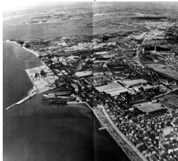
Figure 5. -Aerial view of the plant during the 20th century (photo modified by the author and taken from the book's withdrawal SENA. 1958)
