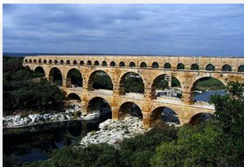
Pict. 9. The multiple arches of the Pont du Gard in Roman Gaul (modern-day southern France). Its lower tiers carry a road across the river, and the upper tiers support an aqueduct conduit that carried water in Roman times
