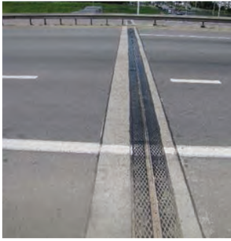
Fig. 11. Minsk ring road, the 8 th km (the joint is installed in 2008).
