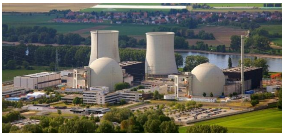
Biblis Nuclear Power Plant, Germany
