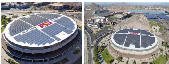
Figure 1.3. Wells Fargo Arena, topped with solar panels
